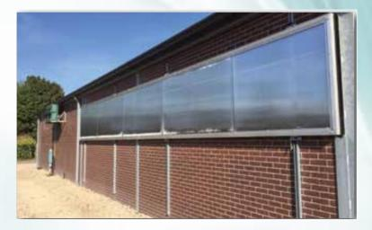
A single-leaf window with polycarbonate filling represents a modular hinged structure on a window opening in a livestock farm. The transparent structure is based on celled polycarbonate (16 mm), which is resistant to ultraviolet. The modules (panels) are up to 2.1 m.
