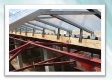
**9. Joining strip** is made of complex aluminum profile (59 mm wide), equipped with a sealing rubber gasket. Installation is carried out with consideration to the compensation of thermal expansion in the place of polycarbonate fastening joint.
