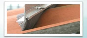
**7. Roof beam –** represents an aluminum profile 66x55x3, installed with a pitch of 1.057 m, with additional rafter stiffeners.
